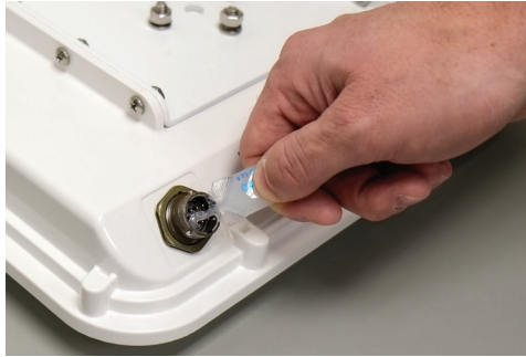
Figure 1.6 – Applying Silicon Dielectric Compound
